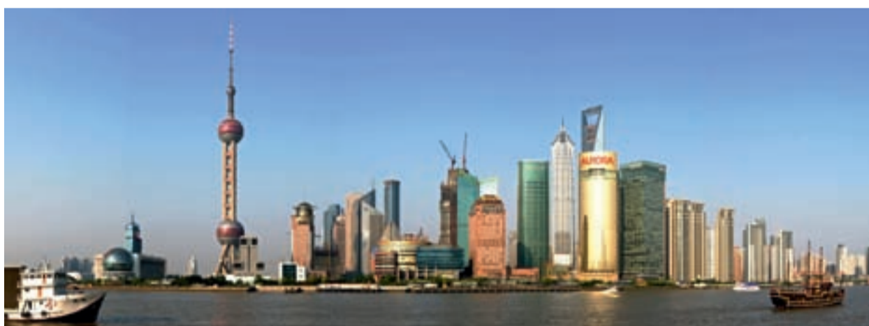
Bauboom in Shanghai
